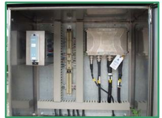
Figure 3: PIU mounted in 11 kV switchgear
