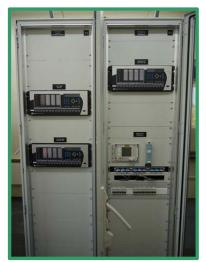
Figure 5: Front view of relay panels
